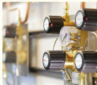
Centralized Gas Supply
